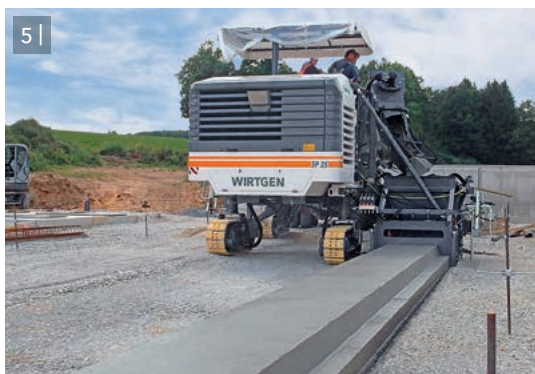
3 | Paving a rainwater gutter with the mould mounted on the left side of the machine.
