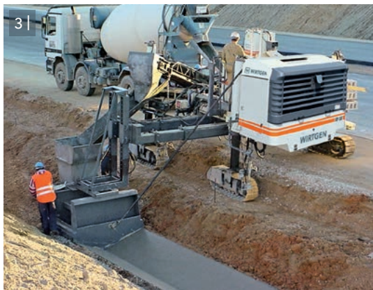
2 | Paving a concrete safety barrier as central reservation.
